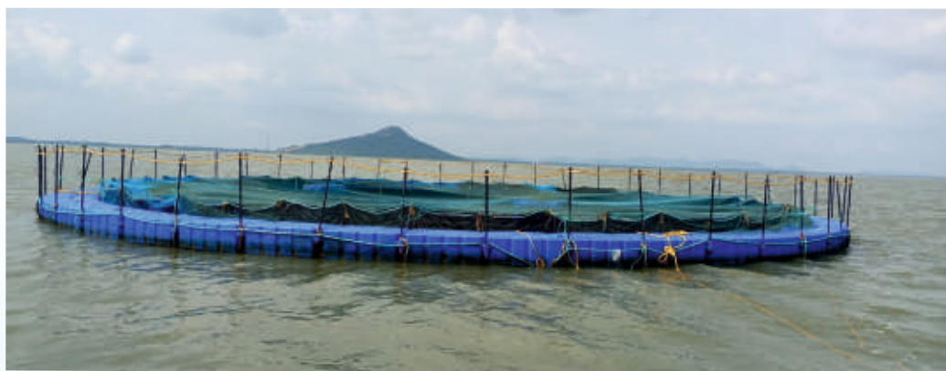
Circular cages installed at the Hirakud reservoir
